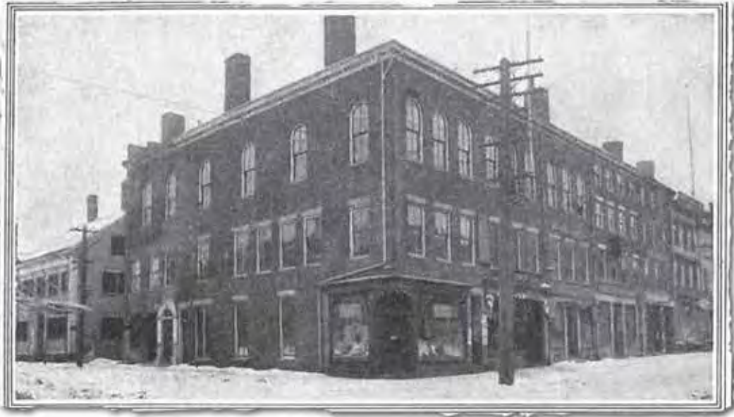
FIRST LOCATION AT THE CORNER OF STATE AND ESSEX STREETS
